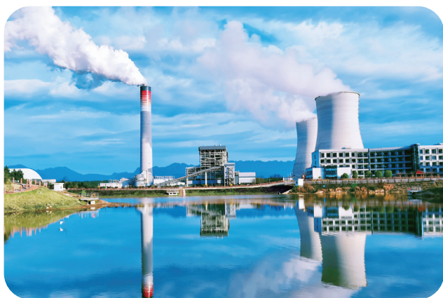
电力行业 Electricity Industry
